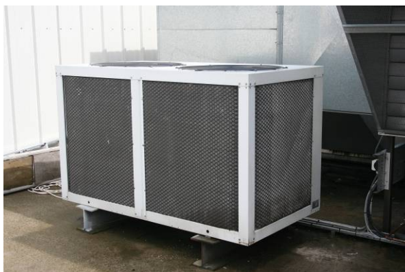
Figure 6 Tecnibel CSAGV -80 air cooled unit
