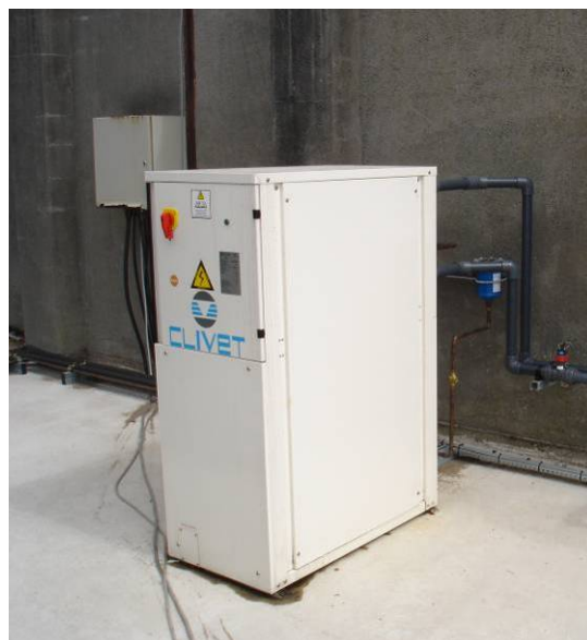
Figure 7 Clivet MCH292 water cooled unit
